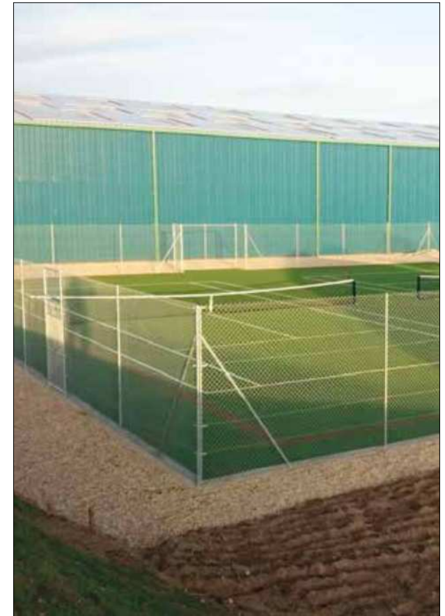
En-Tout-Cas are among the UK's most experienced providers of synthetic sports facilities.
